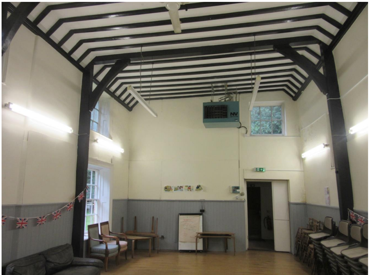
Figure 23: The interior looking south.
