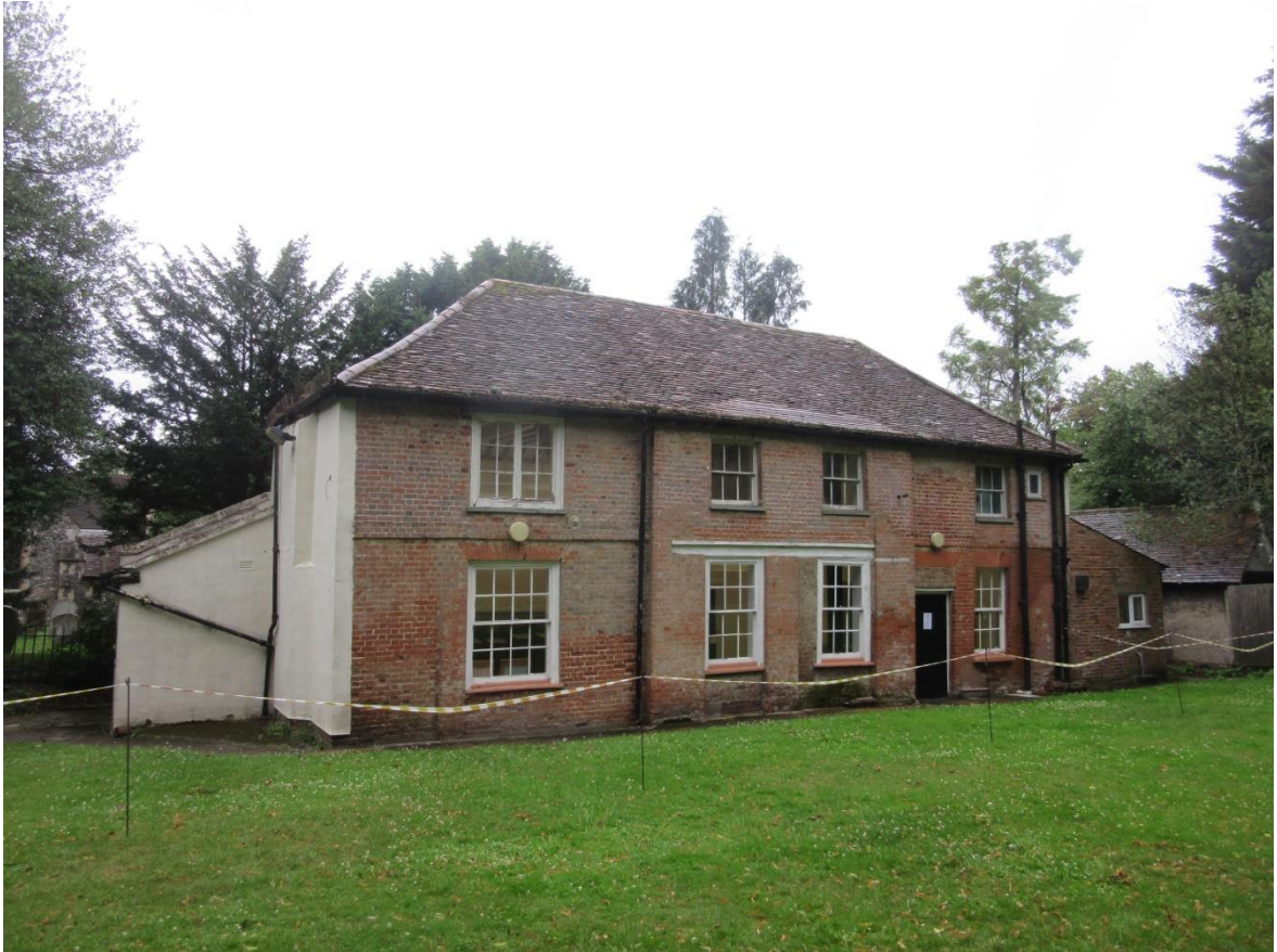
Figure 20: Front (east elevation) of Church House).
