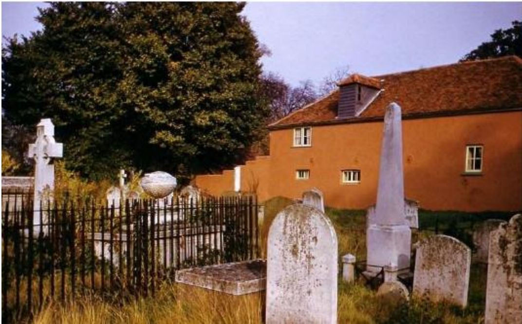
Figure 17: The rear elevation of Church House from the churchyard (c.1960s-1970s).
