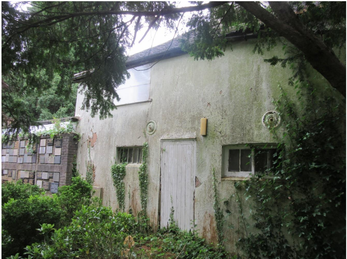
Figure 22: Rear (east) elevation of Church House.
