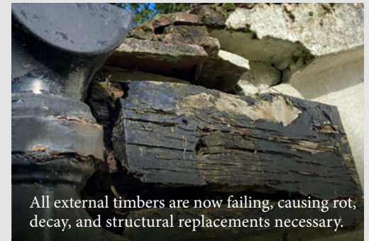
The entire roof structure needs urgent attention. Replacement of framework and tile coverings.
